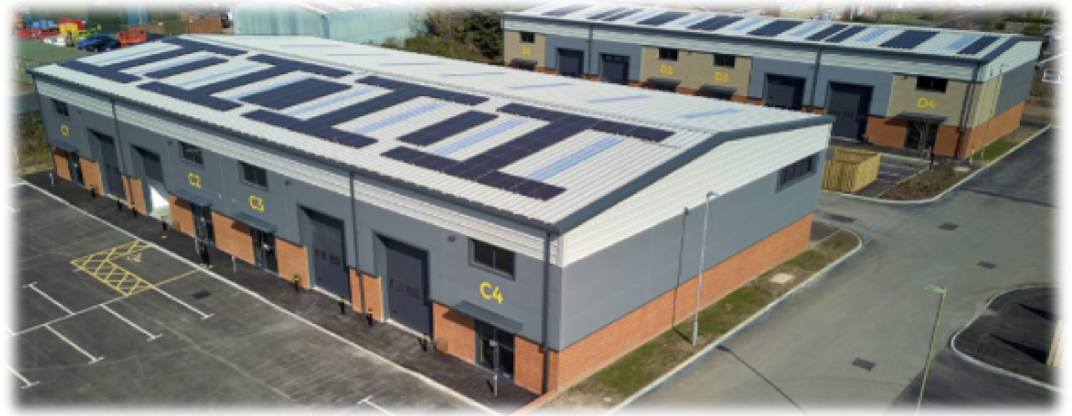
PV roof panels to Blocks A, B, C and D
